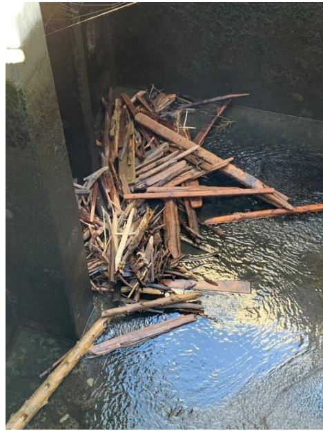
Figures 1 & 2. Large woody debris mat in the flow control section of the South Fish Ladder.
