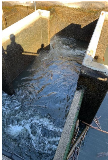
Figures 3 & 4. Large wood debris in the South Fish Ladder with the potential to stop fish passage.
