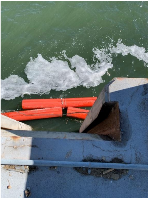
Figure 7. The first temporary debris boom installed on April 20 th , 2021.
