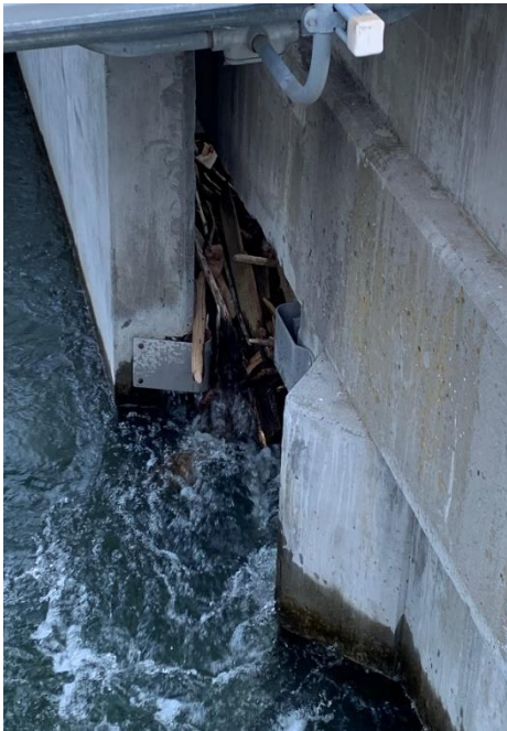
Figures 3 & 4. Large wood debris in the South Fish Ladder with the potential to stop fish passage.
