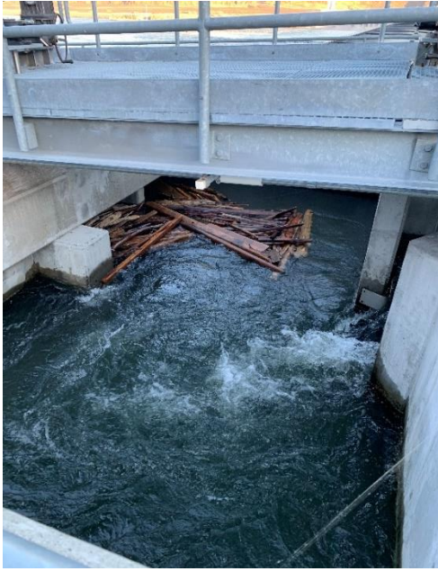
Figures 1 & 2. Large woody debris mat in the flow control section of the South Fish Ladder.
